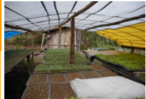
Construction of low cost greenhouses in La Esperanza
