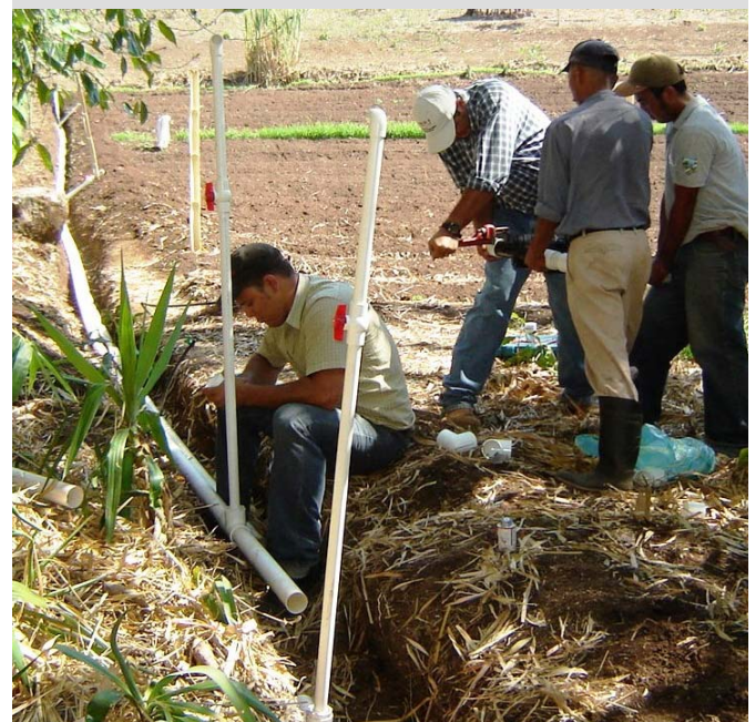
Installation of drip irrigation system, Intibucá
