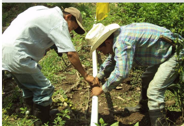
Farmers install a drip irrigation system, in Lempira.
