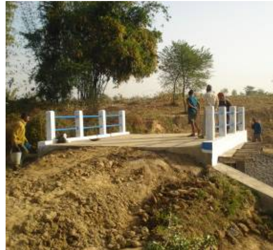
Villagers in Banke walk across a bridge built with USAID-NFRP support.
