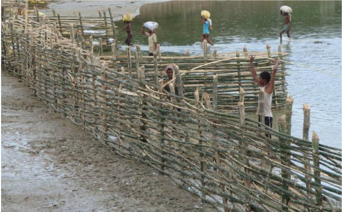
Villagers work to build a river embankment in Barainiya VDC, Bara district.
