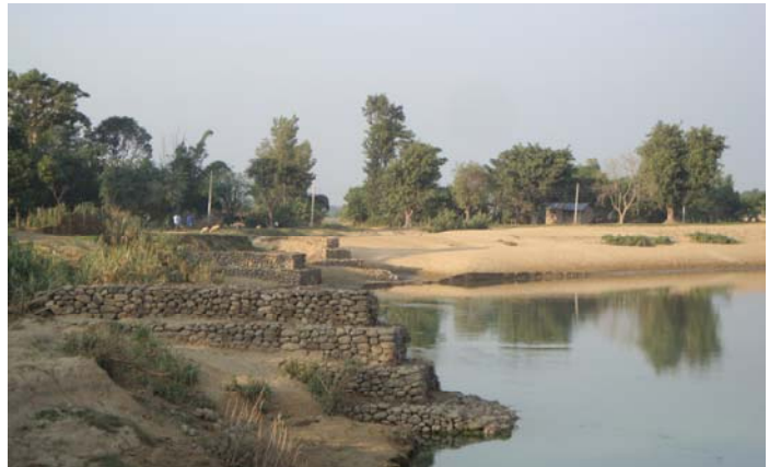
Gabion Box, Basbani village, Joshipur VDC
