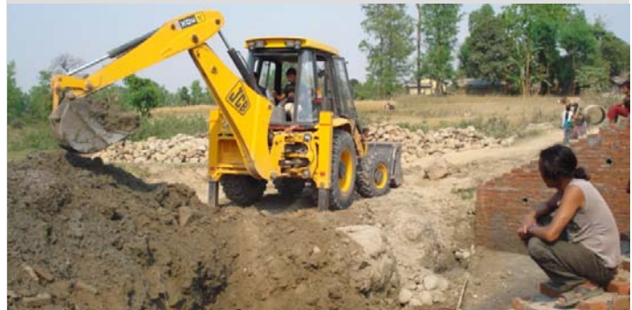
Excavator reshapes roadway – Pachim Kusuha VDC
