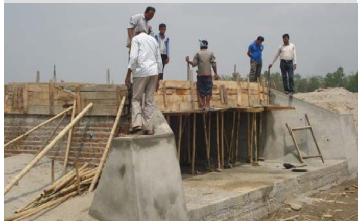
An 8 meter slab culvert nears completion – Haripur VDC
