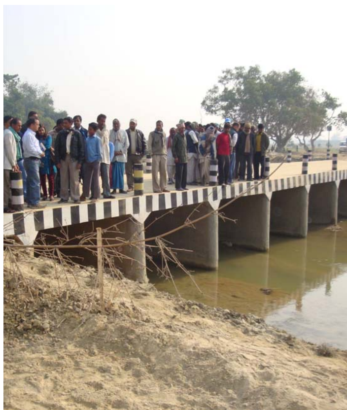
USAID technical staff inspect the large vented culvert constructed by USAID-NFRP in Jaymanglapur VDC (Parsa) during a field monitoring visit.
