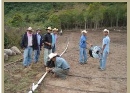
EDA demonstrates drip irrigation installation.
