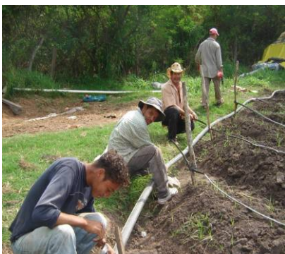
Drip Irrigation Installation
