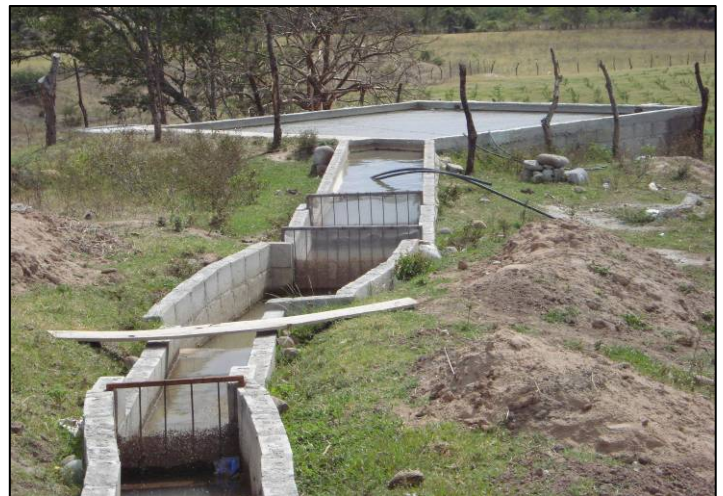
Water reservoir and channels
