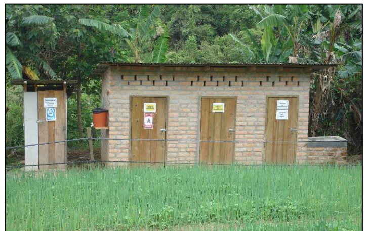
Farm toilet, input/equipment storeroom and washing station
