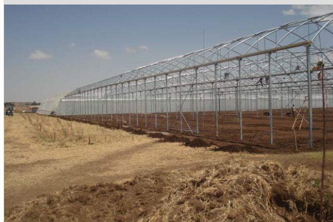
Photos by Fintrac Inc. A greenhouse during construction at Chancho Flowers.
