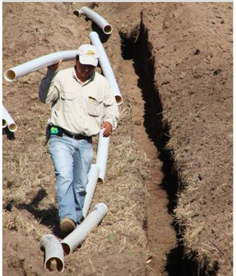
Installation of an Irrigation System in Olanchito.
