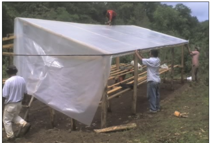
Construction of Greenhouse for Group in Marcala, La Paz
