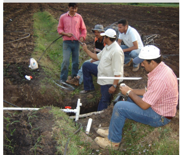
Irrigation system installation, Azacualpa, FM.
