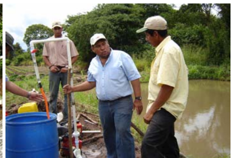
Irrigation System Installation
