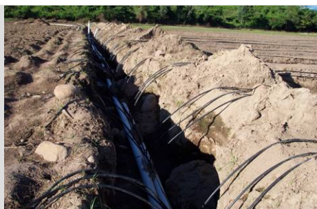
Installation of Irrigation Systems
