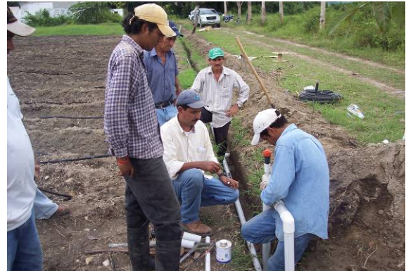
Installing drip-irrigation, Choloma
