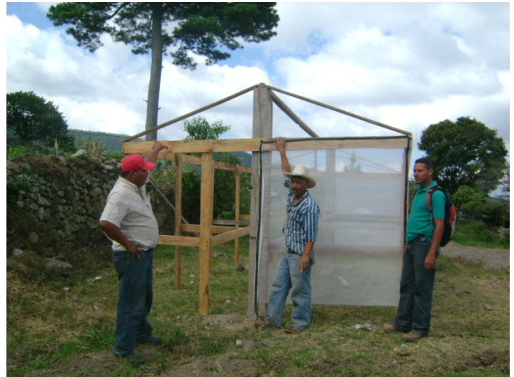
Greenhouse construction with FUNDER producer, Azacualpa, Francisco Morazán
